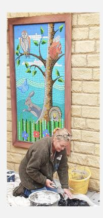
Installation was direct to an exterior wall with a render base and a wooden frame.
